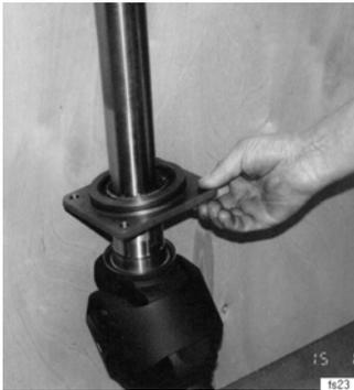
Picture 32 Installation of the drive shaft flange.
